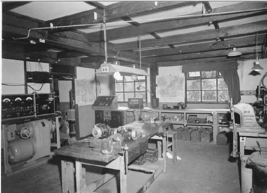
Electric Shop. Starters, generators, inverters, and conduits are just a few of the items repaired in volume by the men in this shop. Among its many accomplishments, this shop, under the direction of T/Sgt Heil, installed emergency power installations for the various shop buildings and machinery. Working with T/Sgt Heil are S/Sgt Ranweiler, Mallery, Barker, Dragoo, Travis; Sgts Brown, Friedberg, and Pray.
