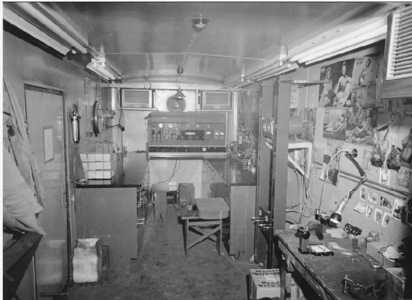
Instrument Shop. This shop is housed in two trailers, and space is limited, but the volume of work is anything but limited. Certain line work is handled by this department. A newly added job is that of checking electronic supercharger regulators. One man is kept very busy all the time taking care of the many watches brought in for checking and repair. M/Sgt Harper is in charge and assisted by T/Sgt Hanson, S/Sgts Burzlaff and Patocka, Sgts Wrigley and Giesing.
