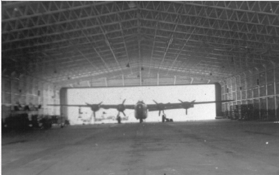
Hangar #1. This is the assembly line of the Sub Depot. New and repaired parts replace damaged parts. Broken hydraulic lines are replaced, wiring repaired, and engines changed. In fact, anything and everything is done in this Hangar to keep a plane flyable. Assisting M/Sgt Joe Napier to "Keep 'em flying" are T/Sgts Mall, Neal, Johnson, Schnieder, Iho, Garlitz, Nolan, S/Sgts Nauert, Maddox, Reed, Bayha, Piekarz, Morrison, Malfe, Macko, Neill, Cygnarowicz, Sgts Nawrocki, Klein, Dietrich, Martin, Urton, Hylton, Dally, Scott, White, Schicchi, Allan, Cpls Stevens, Ulstad, Kaylor, Spiegel, Smith, Pfc Zeiga, Gomez, Leibowitz, Holt and Barnes.
