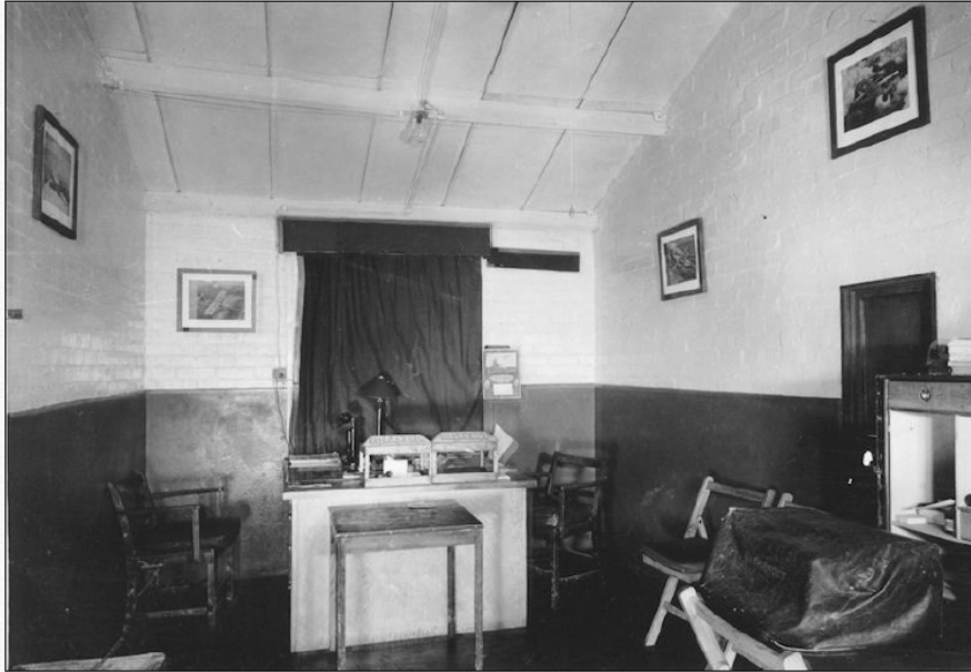
Office of the Commanding Officer and the Sub Depot Supply Officer. The Commanding Officer's and the Sub Depot Supply Officer's office is where all the major problems are solved and major decisions are made.
