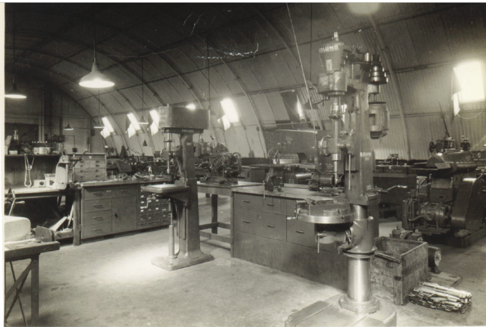
GE-122-42-392X4-9-44 (SUB-DEPOT) Machine Shop. This shop has expanded from a one-lathe trailer to a full-sized shop with four lathes, milling machine, shaper, Do-All machine, power hacksaw, and other necessary machinery to do any job required. This shop has 14 machinists: T/Sgt Tevlin, Department head, T/Sgt Girard, S/Sgt Kay, Casale, Mahan, Neville, Sgts Jones, Clark, Cpls Hageman, Nuccio, Burke, Montross, Pfc Sedor and Pvt Wortman.
