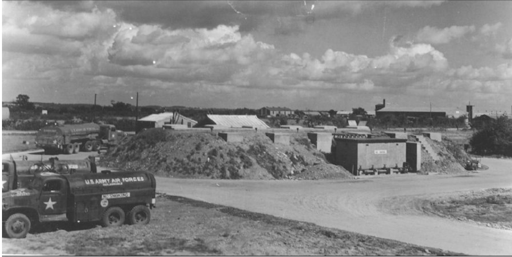
Petrol Installation No. 2. Composite view shows complete installation. In center front is view of one of the two pump houses. Partially-covered cement pillars are bomb vaults. Last building center left is Picket post in which Gas Dump personnel are quartered. The capacity of this installation is 72,000 Imperial Gallons.
